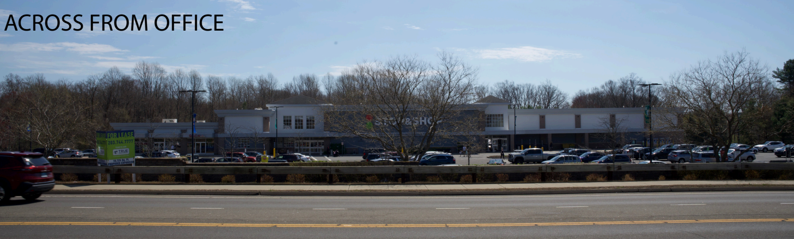
FRONT OF OFFICE
